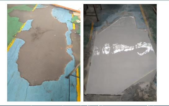
گ Damaged Concrete Floor Rebuilt with Duromar DuroFil Protected with Duromar DF-1310
