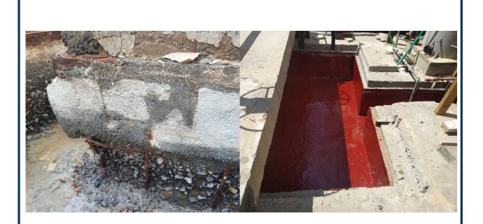
Damaged Acid Neutralization Trench Rebuilt with Duromar DuroFil & Protected with Duromar DF-4301
